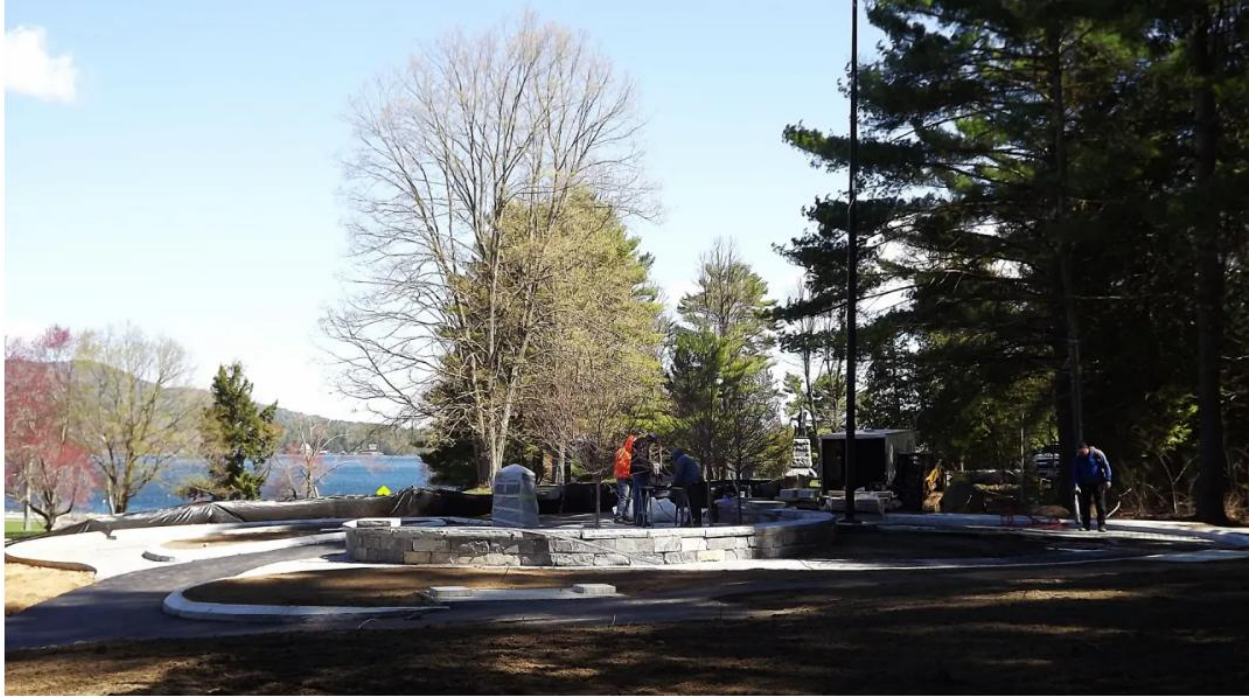
Construction of the memorial plaza on Fort George Road began in October 2025.
