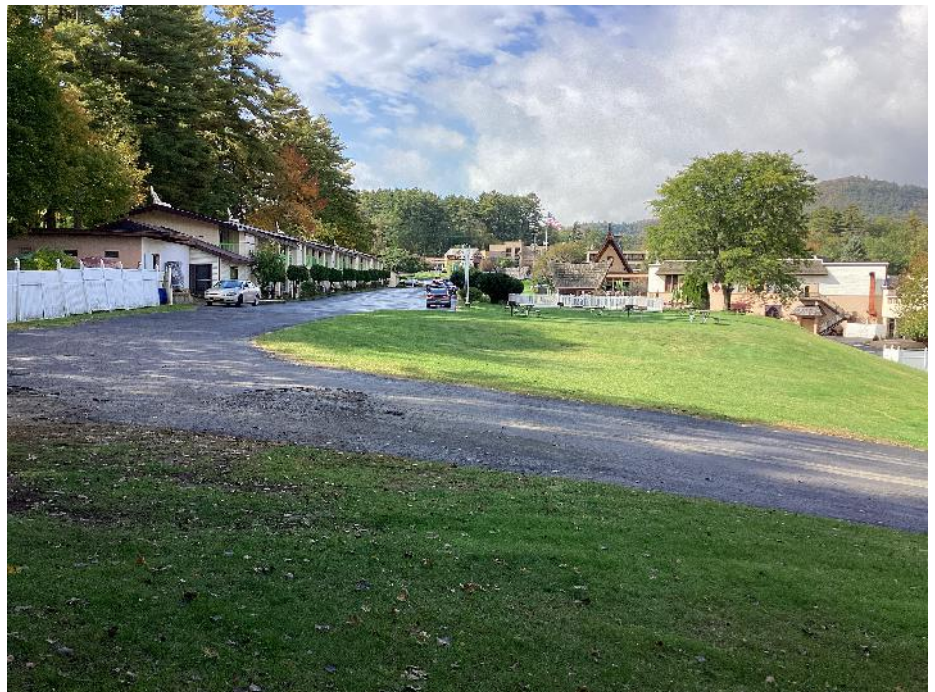
Figure 10. View looking toward Route 9 with Tiki driveway in foreground and picnic lawn in center. Slope at right and driveway drop down to parking lot. Photo taken from area of fill above historic “Gully No. 3.”
