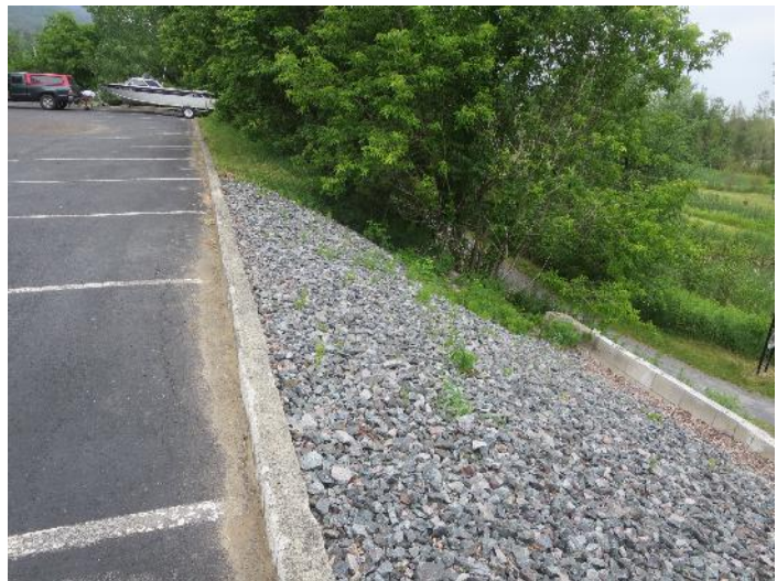
Figure 8. Tiki parking lot sits on approximately ten feet of fill above original marsh.
