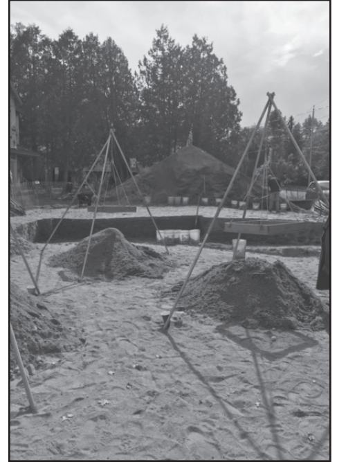
The pile of sand from the excavation was 25 meters long and 5 meters wide and initially started approximately where the most distance sifter is located.
